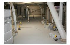
Every silo now has a VEGAPULS 69 that replaced the existing silo weighing system.
