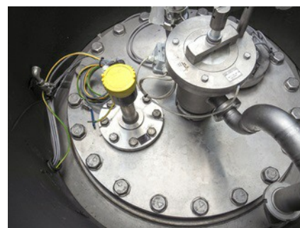
A VEGAPULS 64 radar level transmitter performs contents measurement.
