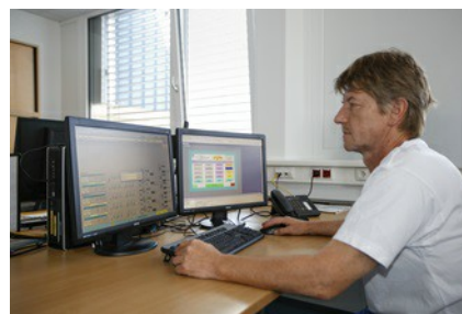
Martin Schneider, master electrician at Berglandmilch, has his eye on all material and energy streams.
