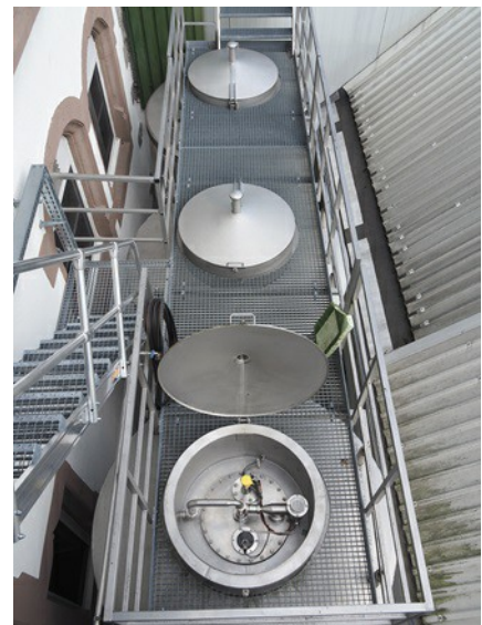
View of a VEGAPULS 63 radar level transmitter on one of the maturation vessels.
