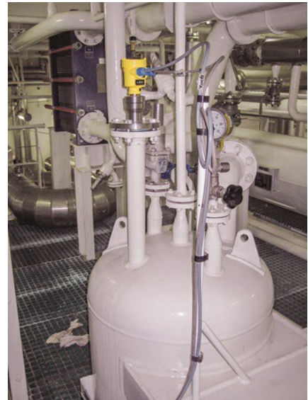
VEGAPULS 64 measures the level in a cooling system on board a gas tanker.
