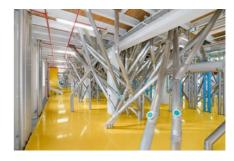
The piping network conveys the intermediate products to the roller mills. Every process step is comprehensively monitored during operation.
