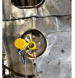
A sturdy 'combination' flange is installed on top of the boiler, it brings two instruments together on one process connection that are essential for the safe process control of the boiler. This transmitter and level switch combination delivers live boiler level information and makes the process more secure, as both instruments can confirm the reliability of each other's results.
