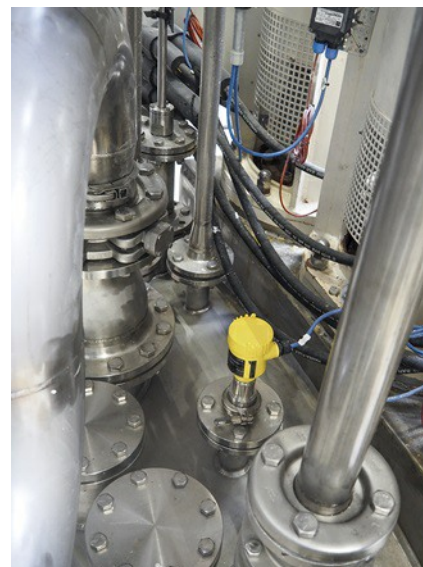
The radar level transmitter VEGAPULS 64 measures the levels in the production equipment with reliability and accuracy.
