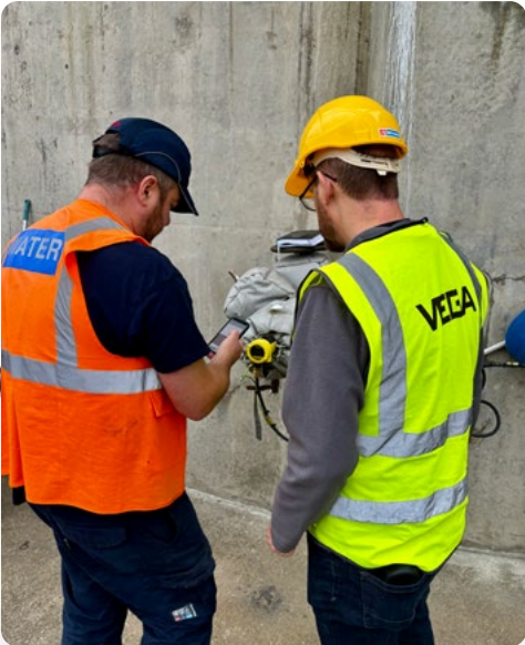
Commissioning a VEGABAR 80 Series pressure transmitter for sludge digester level measurement, supporting reliable operation and efficient wastewater treatment.
