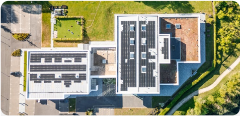
Photovoltaic system: VEGA UK
