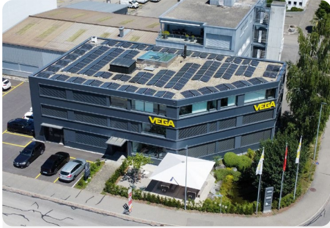
Photovoltaic system: VEGA Switzerland
